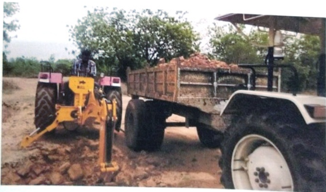
Fig 8. Field Test – Digging & Loading
