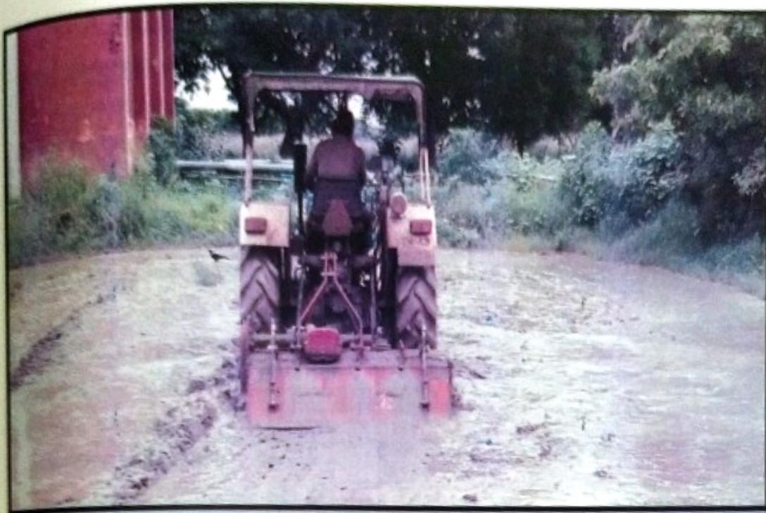
Fig.6. Field Test – Wet land
