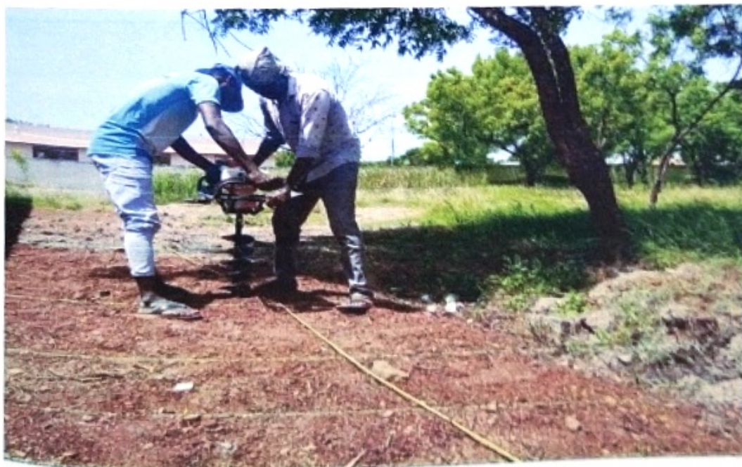
Fig.1. Operational view of the Post hole digger
