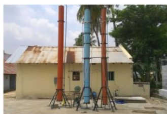
Biogas scrubbing columns with splash tower
