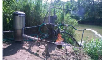
Gasifier- Water Pumping
