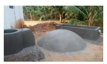
Night Soil cum Kitchen Waste based Biogas Plant is the integration of modern biogas technology with disposal of night soil and food wastes generated from hostel kitchens and dining halls for harnessing bio-based energy.
