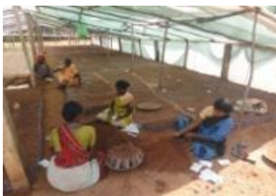
Workers active in preparation of pot mixture
